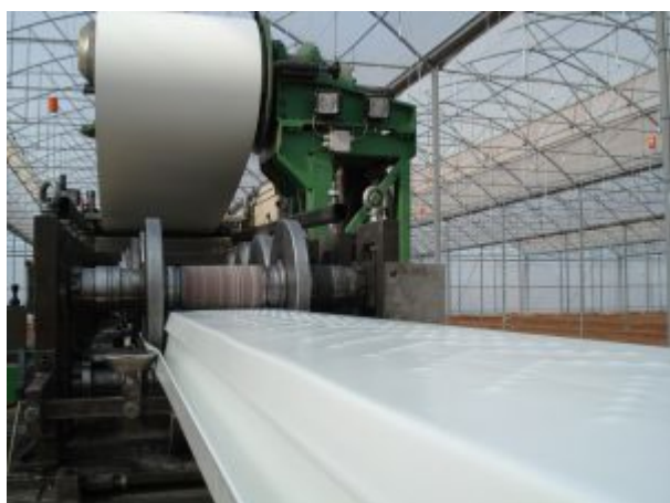
Rolling out gutters inside a greenhouse
